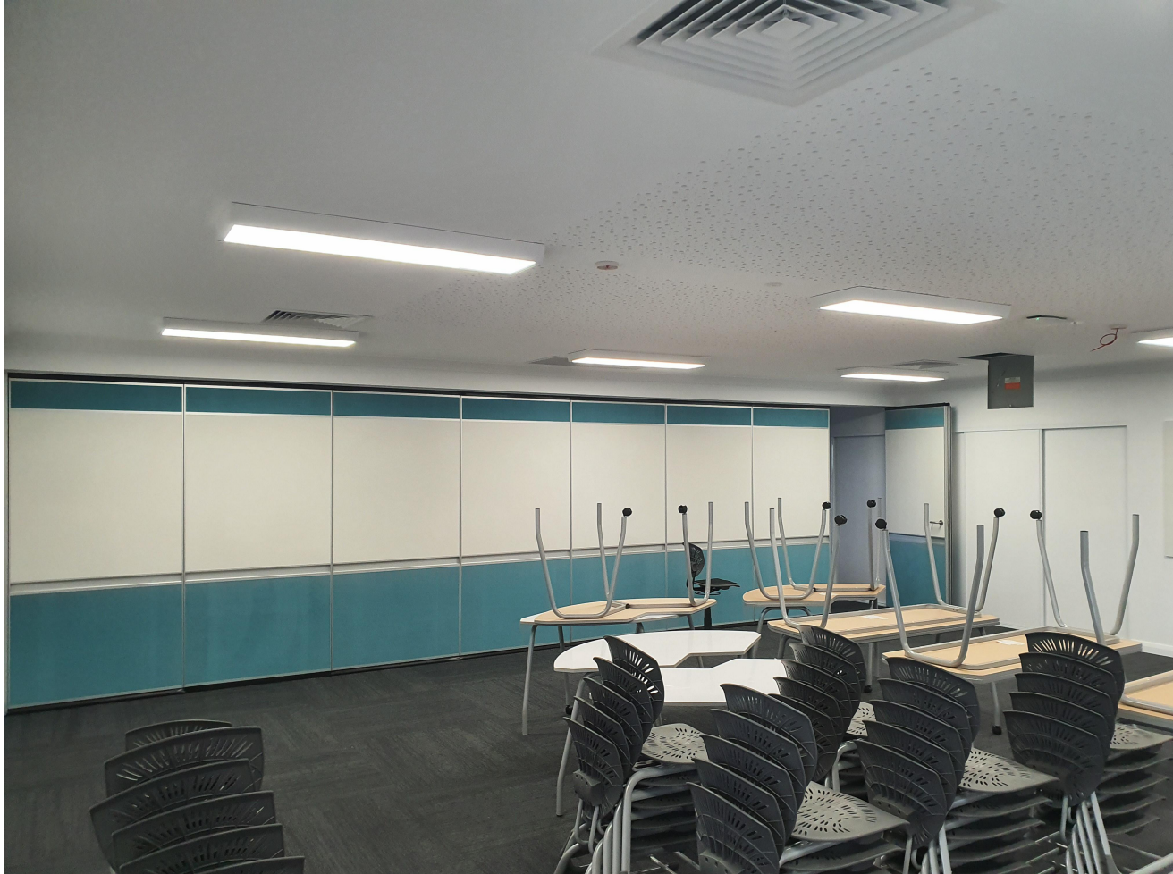
PROPOSED OPERABLE WALL WITH PASSTHROUGH PANEL - AUTEX & WHITEBOARD SURFACE FINISH
