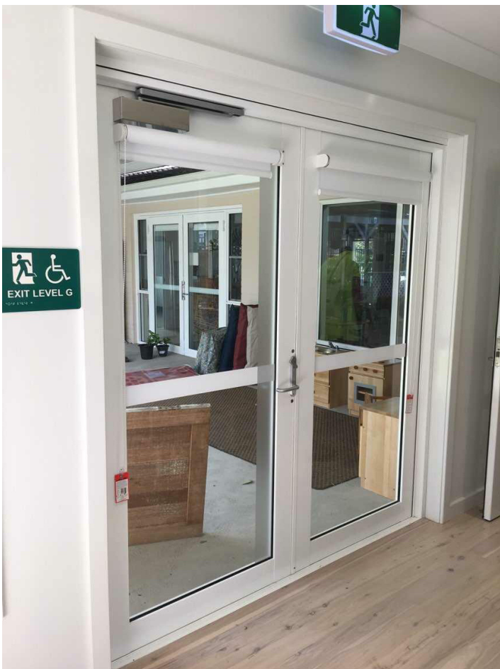
EXAMPLE: ACCESSIBLE ENTRY DOOR WAY - INDICATING EXIT SIGNS, GLAZING MOTIFS & ROLLER BLINDS
